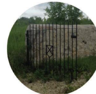
wrought iron fencing
