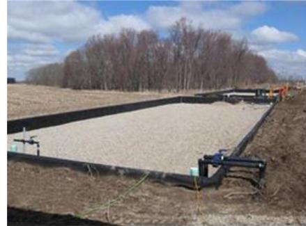
In addition to providing oxygen for nitrification the proposed aeration system brings numerous other long-term performance benefits to this sub-surface flow system.
