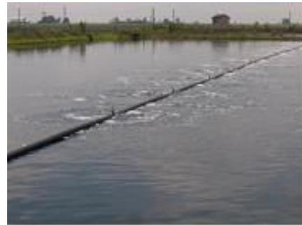
Laterals connect to the shallow buried header, and float on the water surface. With floating laterals, there are no concrete weights required to be in contact with the bottom of the basin. Laterals are secured against wind action with a stainless steel cable system. The cables are fastened to anchors in the berm using a self-adjusting lateral tensioning assembly.
