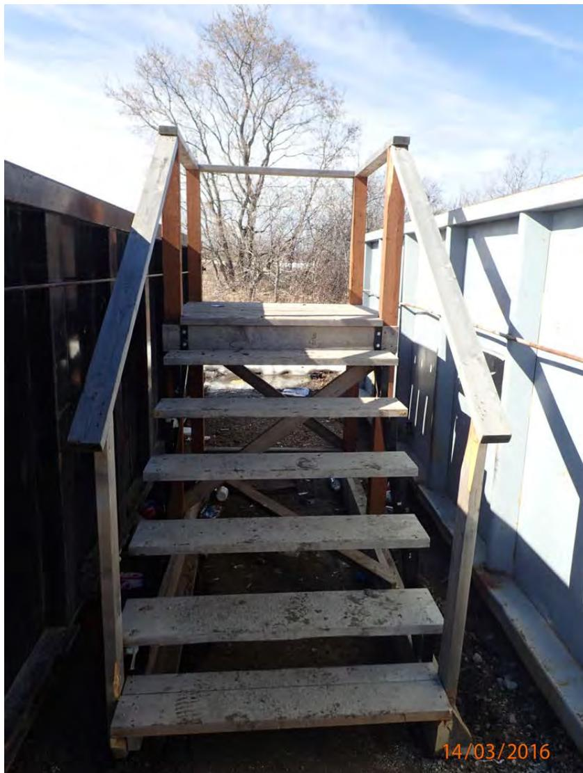
One challenge is that these containers are 6 to 8 m long and the platforms are, at most, 1.2 m in length and are not movable by the public. To ensure proper distribution of the products in the bin, the customer is required to throw their recycling upwards of 4 m from where they are standing.
