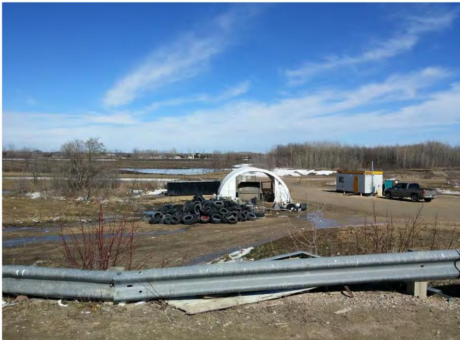
*Guardrail is well below OH&S height requirements (under 1.1 m)*
