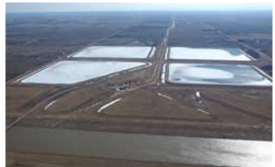
Figure 2 – Aerial view of Deacon Reservoir
