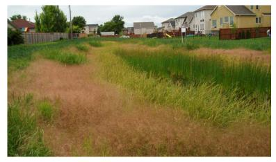
Bio-swale, Seven Oaks subdivision, Winnipeg, Manitoba. Bio-retention systems are designed to mimic processes that occur in the natural environment by filtering and storing runoff water from rainstorms and snow melt, rather than letting it be flushed through the stormwater sewer system.
